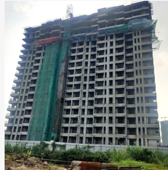
ORCHID - 18 SLABS COMPLETED
