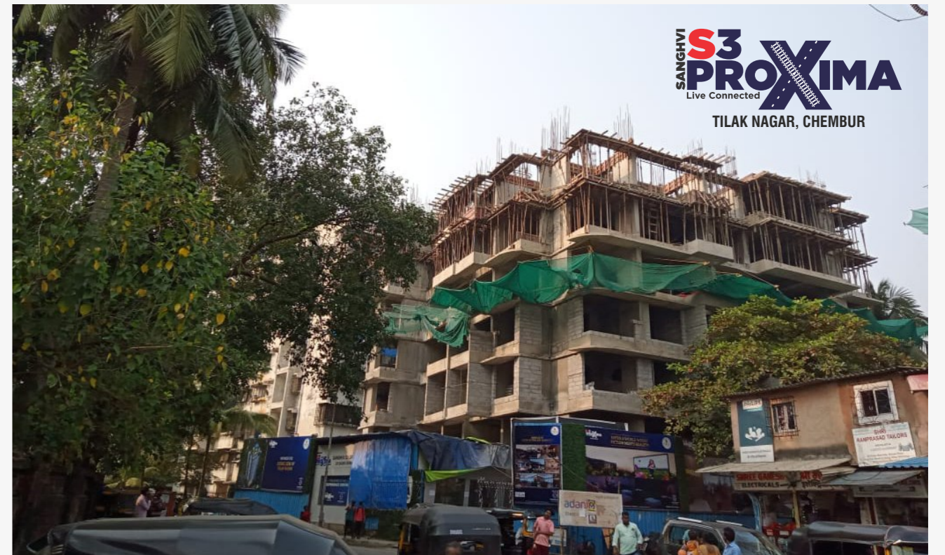
PROXIMA - 6TH SLAB IN PROGRESS
