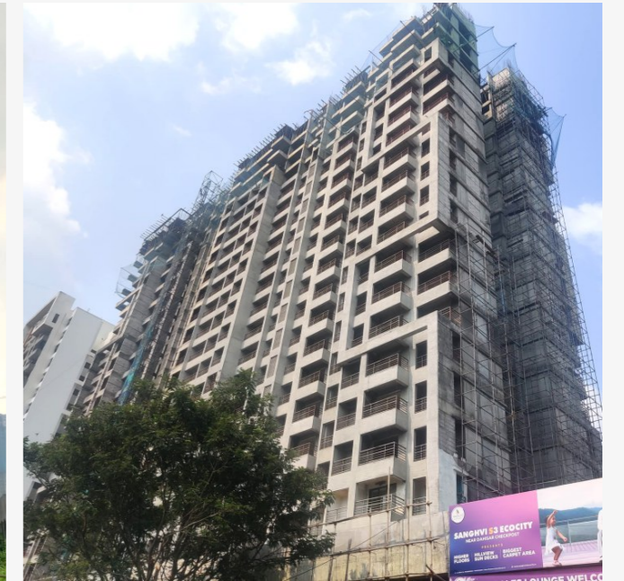
WOODS - 20 SLABS COMPLETED
