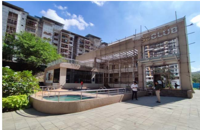
Completed Club House
