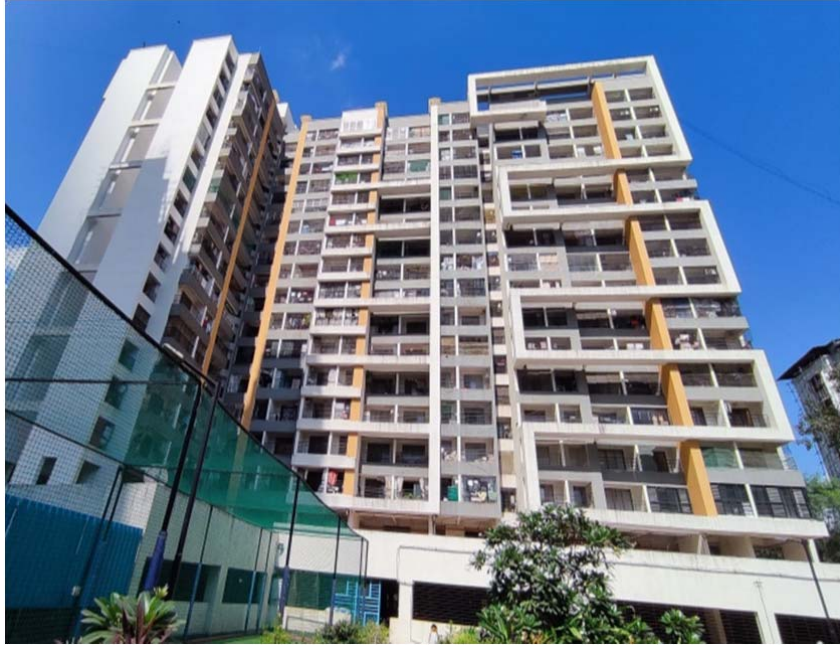
Plot A: Completed Bldg. No. 5, 6 & 7
